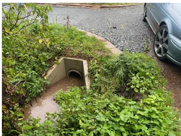
Photo 1 – Drain to take water from Turners Lane
